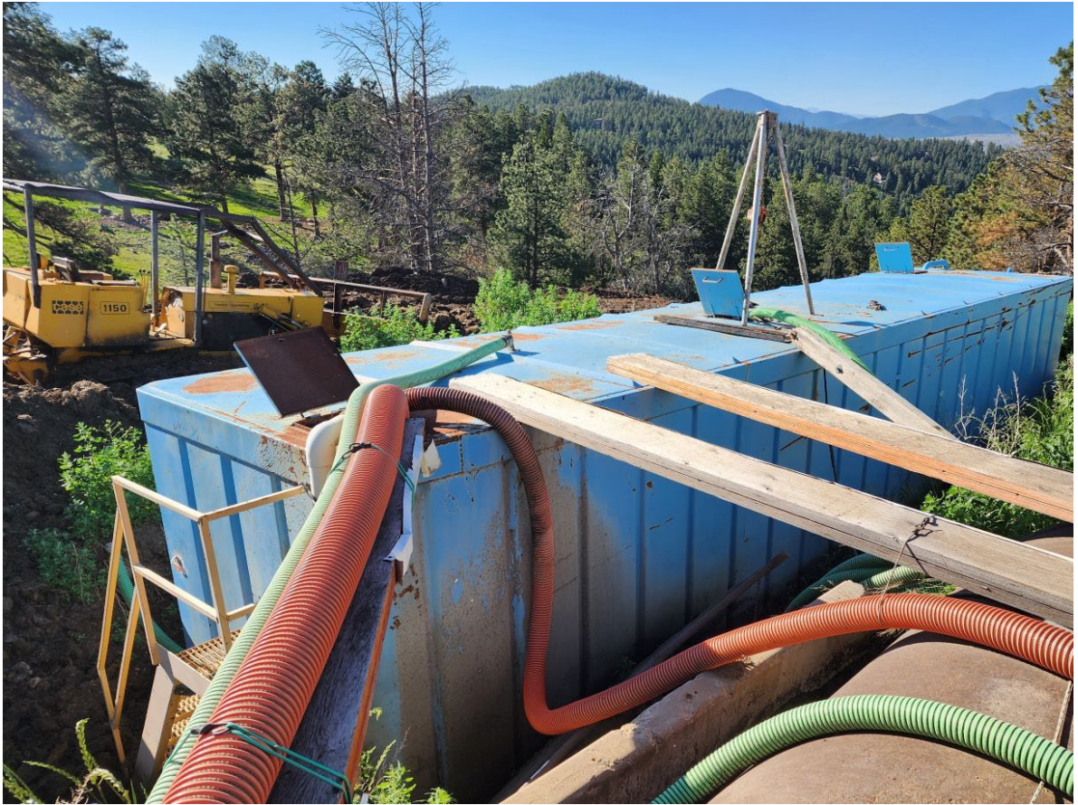
Photo 3: First frac tank that receives septage after pH adjustment and screening.
