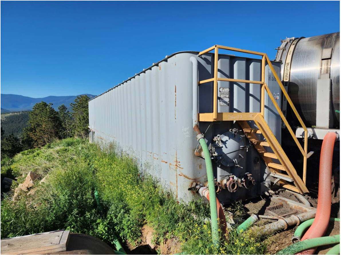
Photo 5: Second frac tank next to dewatering unit.
